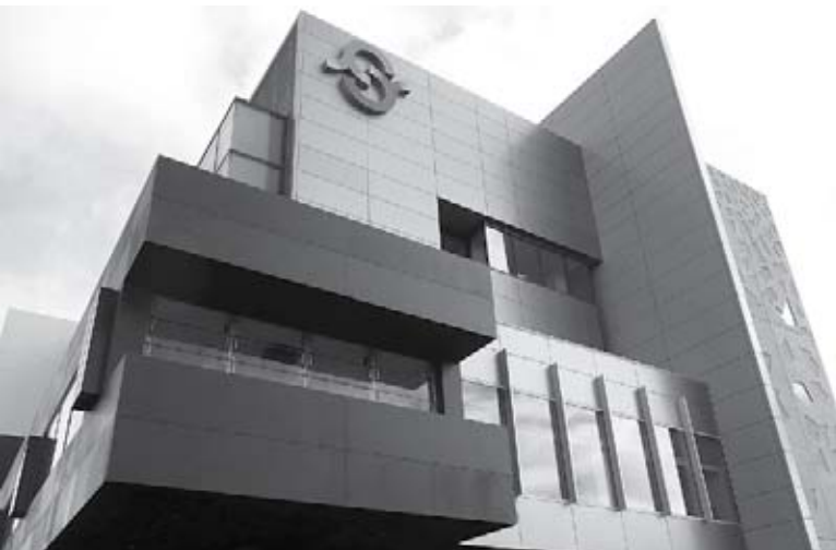
Our new $115 million Warrnambool Base Hospital.
