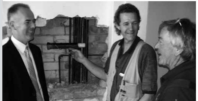
SWH carpenter Lindsay Hess (centre) and plumber James Moran show CEO John Krygger the time capsule.
