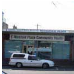
Manifold Place Manifold Street Camperdown 3260 ph. (03) 5593 1892 fax. (03) 5593 2010
